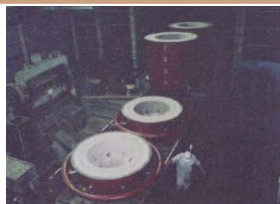
Fire-resistant furnace for electric power generation Interior: refractory brick insulated
